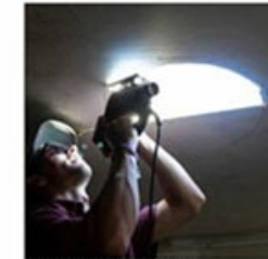
CUTTING HOLE IN RESIDENTS ROOF
