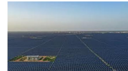
Bhadla Solar Park:
